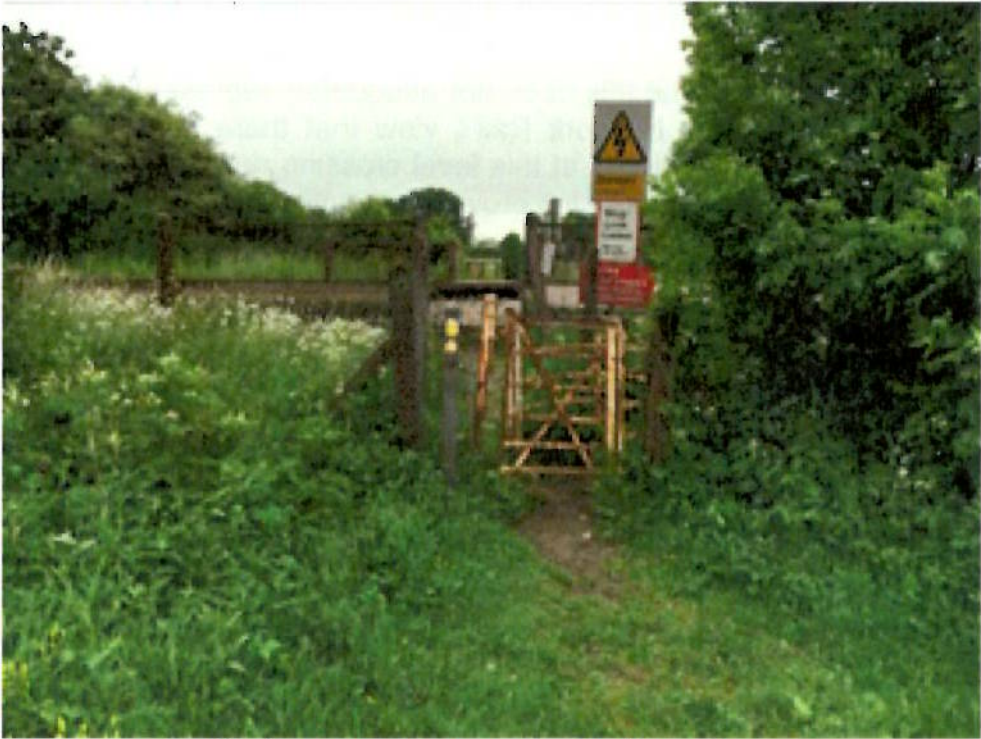
Level crossing kissing gates from north of railway line
