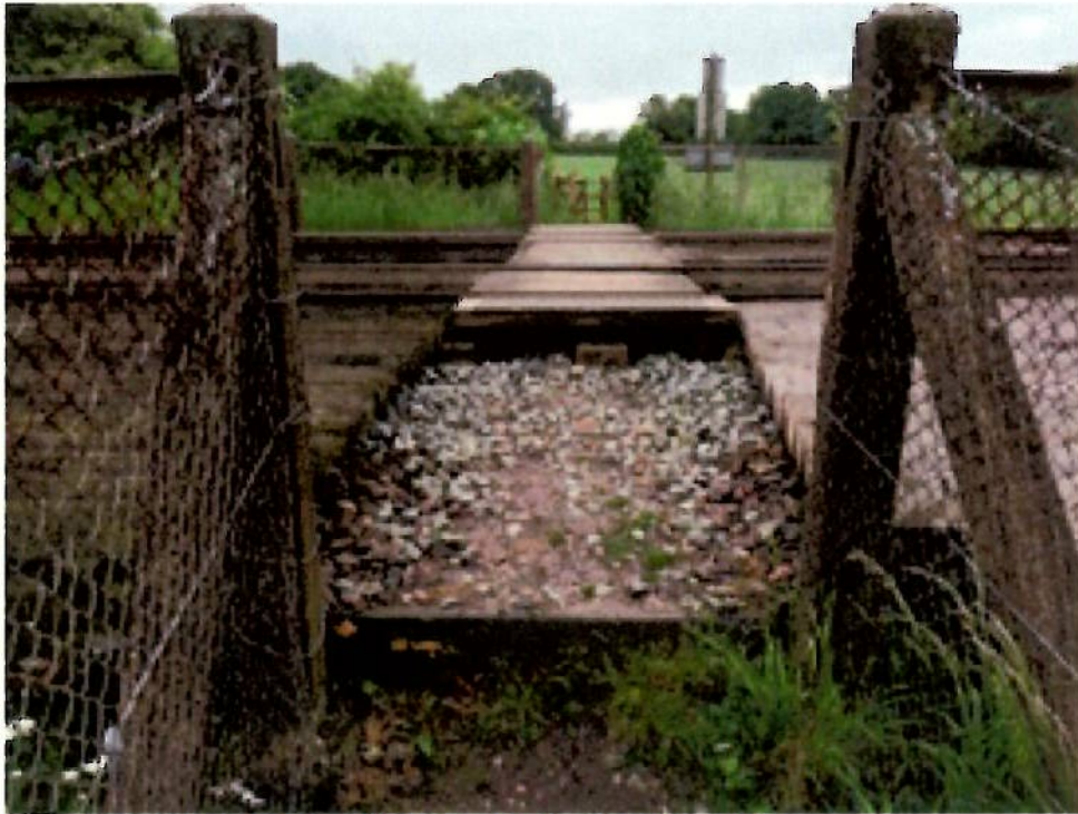
Level crossing approach from south of railway line
