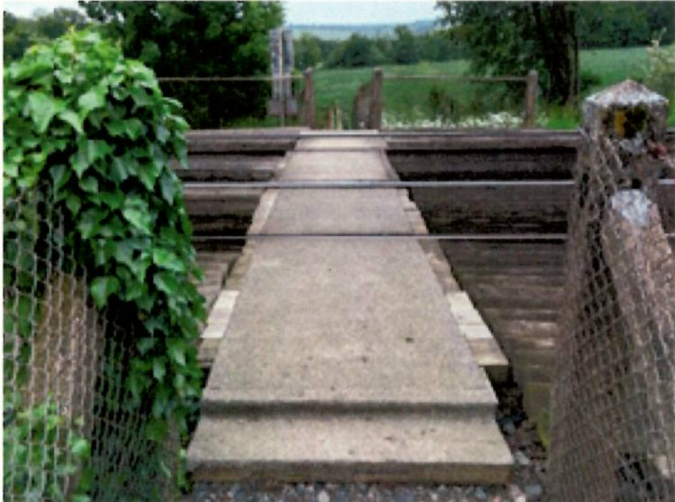
Level crossing approach from north of railway line
