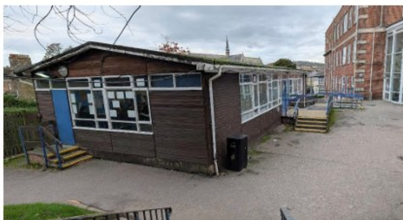
Area B – existing mobile classroom
