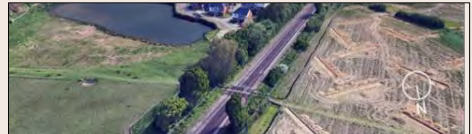
Figure 12 - Cradle Bridge Crossing
