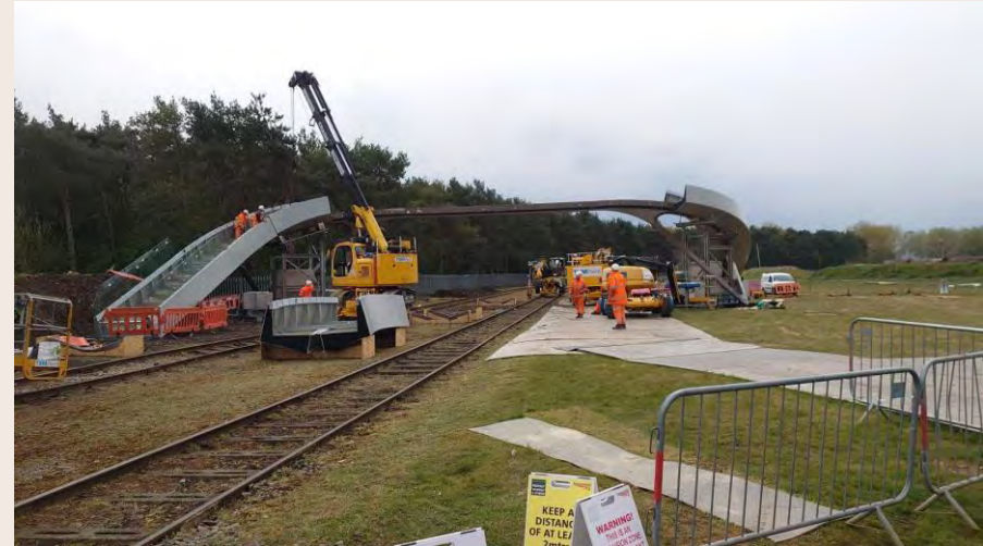
Flow Bridge Mark 1 installation photo – Stair FRP units
