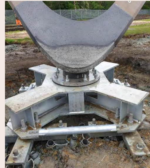
Rapidroot system installation photo
