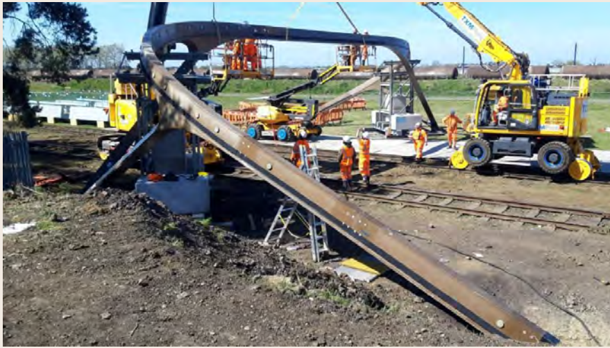
Flow Bridge Mark 1 installation photo – Spine
