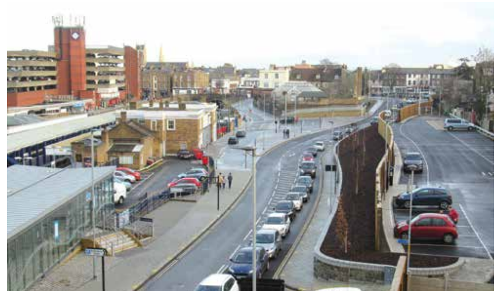
Rathmore Road completed improvements in Gravesend
