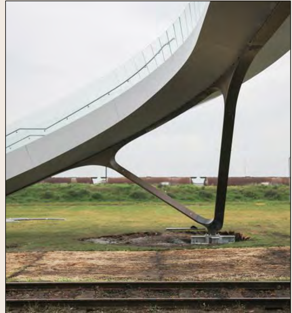
Figure 5 - Flow Bridge pier
