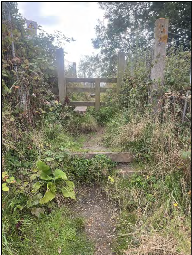
PHOTO 2: PEDESTRIAN STILE TO DOWNSIDE SHOWING STEPPED ACCESS
