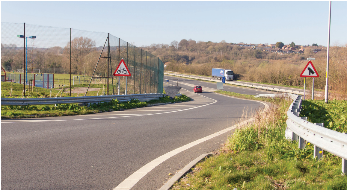
Figure 1.2 A2 London Bound On-Slip Road
