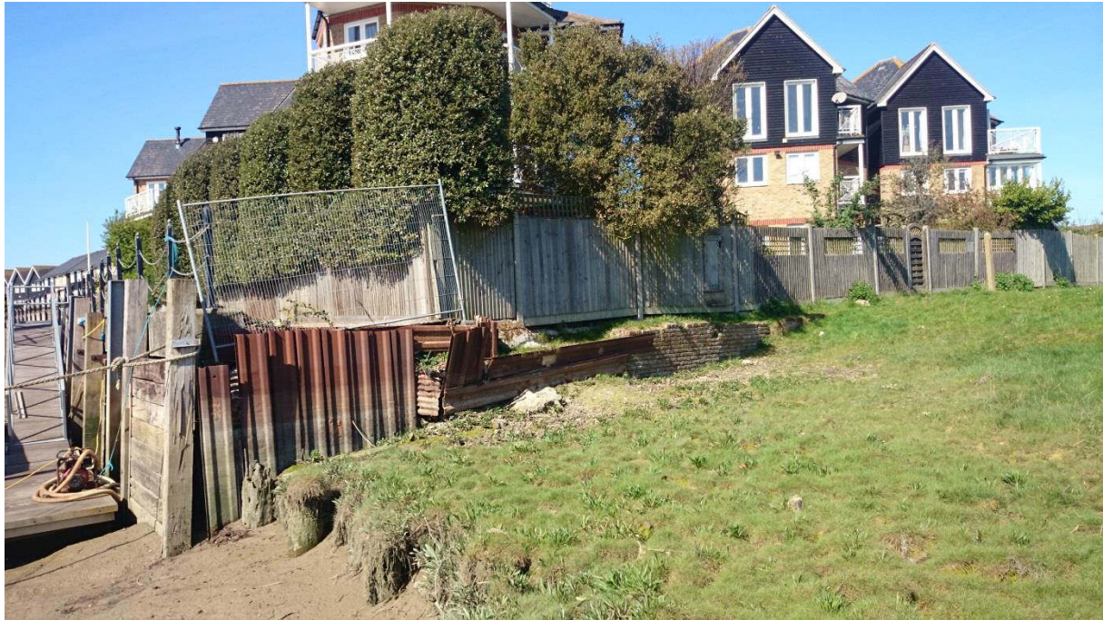
Photograph 11: View of location L-M looking west.
