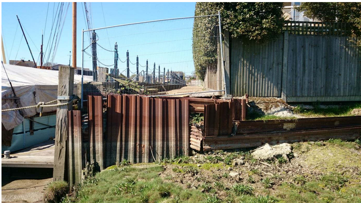
Photograph 10: View of location L-M looking west.
