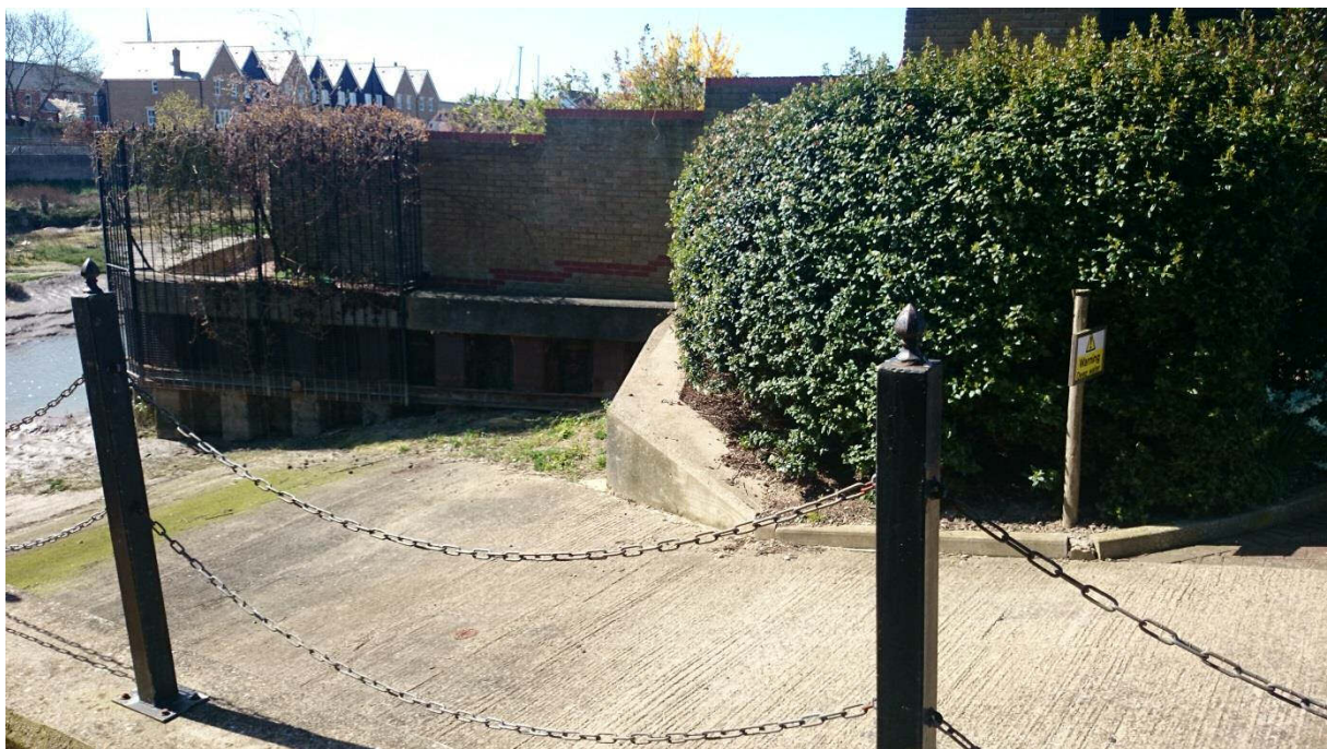
Photograph 8: View of location H-I looking west.
