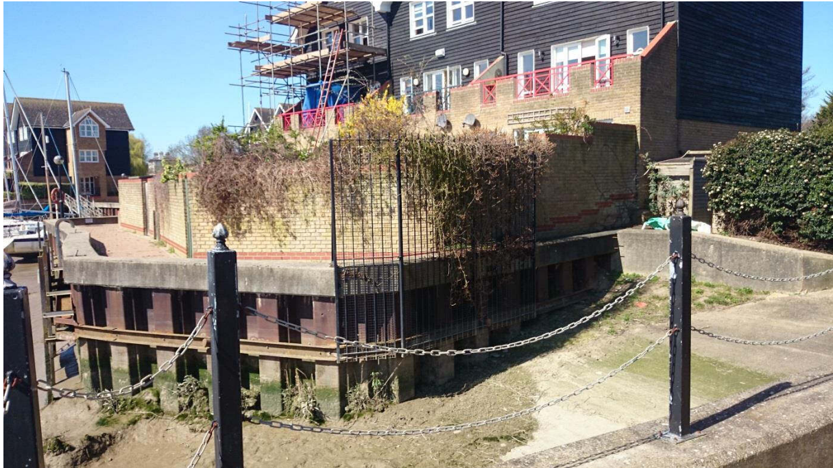
Photograph 9: View of location H-I looking west.
