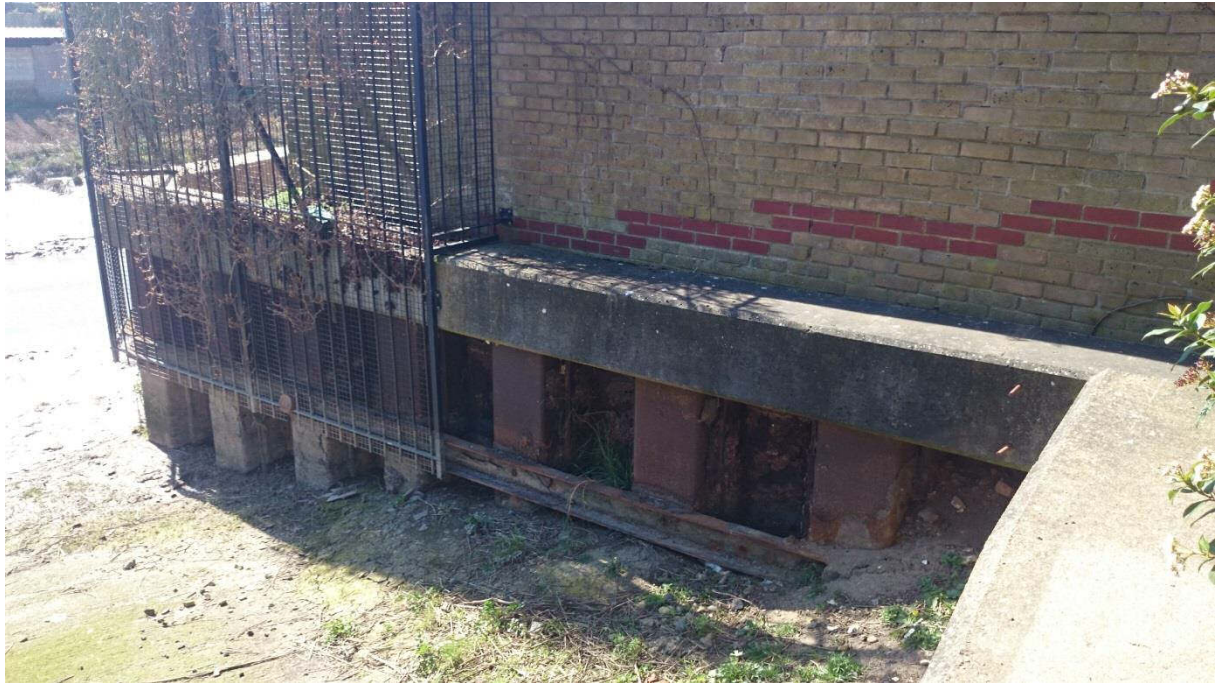
Photograph 7: View of location H-I looking west.
