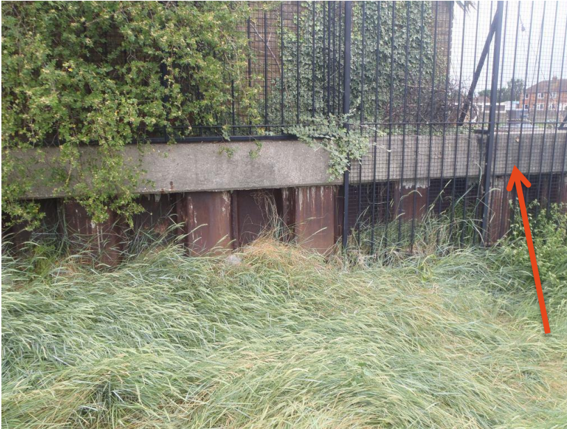
Photograph 1 – Showing proposed ramp location at point B (see red arrow).
