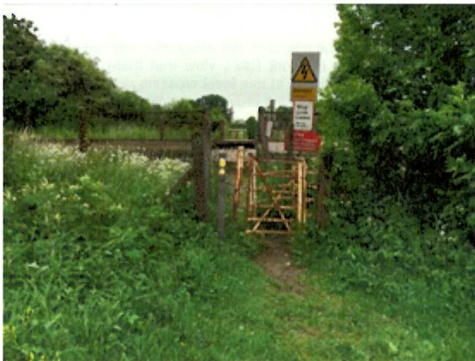
Level crossing kissing gates from north of railway line
