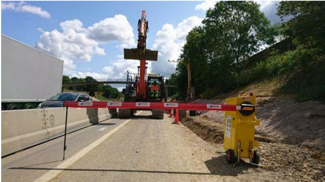
The UK's first solar hybrid, instant deployment, work zone protection vehicle barrier
