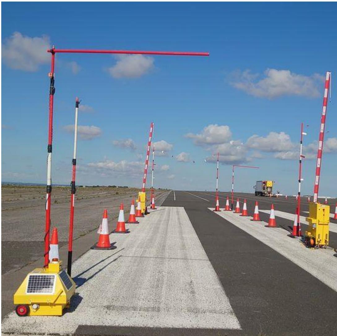
The INSTABOOM GS6 barrier is specially designed to protect against overhead strikes in work zones
