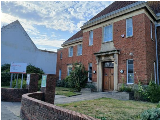
Miscellaneous Assets include assets such as land next to highways, buildings not used by KCC, specialist PFI sites and vacant sites for disposal/Alternative use.
