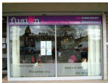
Fusion Healthy Living Centre received £7000 towards refurbishment
