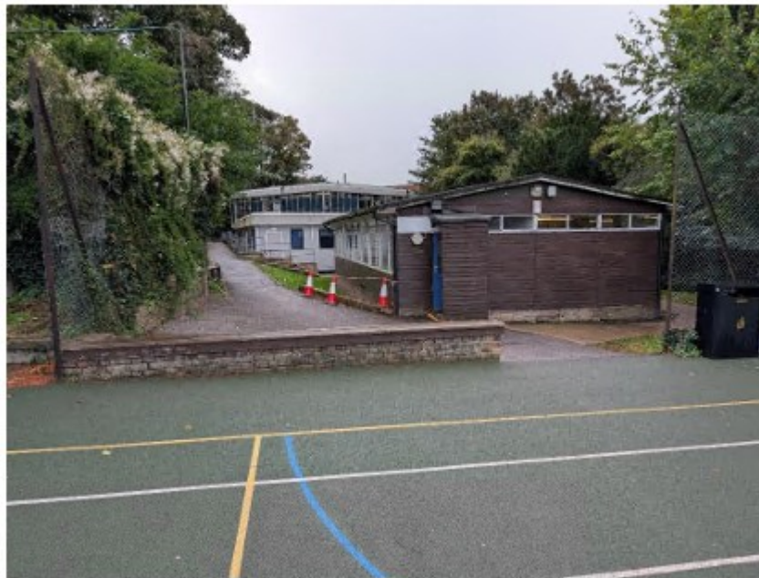
Area A – Mobile F – existing mobile classroom
