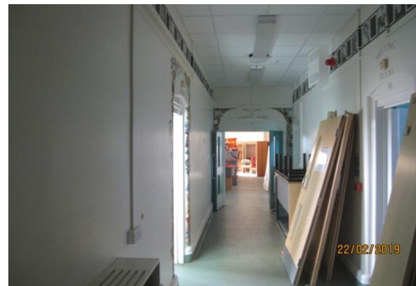
Ramsey Ward Entrance (Not in Use)
