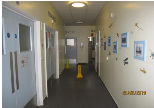
Cranmer internal corridor
