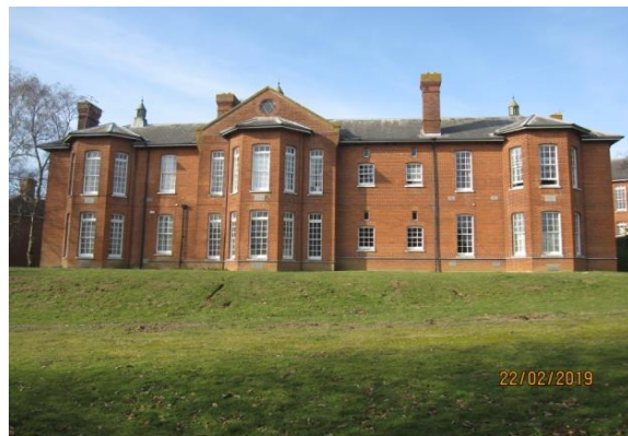
One of main ward blocks not in use
