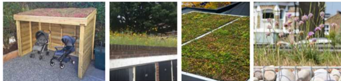
③ New buggy stores and bin stores with green roofs for water management and wildlife benefit.
